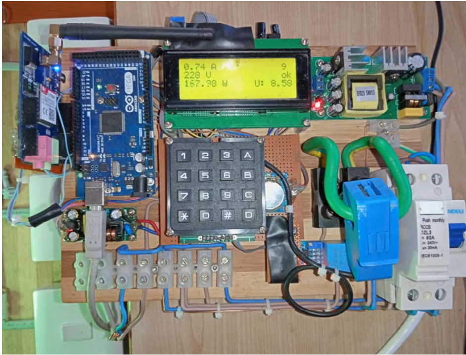
Fig.5. Smart Meter Unit During Testing
