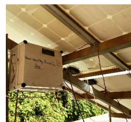
Fig. 4. Solar panels with Zigbee
