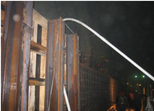
Figure 4. Crane beam on rock wall in construction
