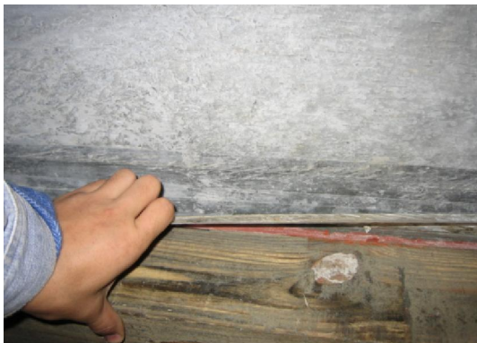
Figure 5. VISA mould of the crane beam
